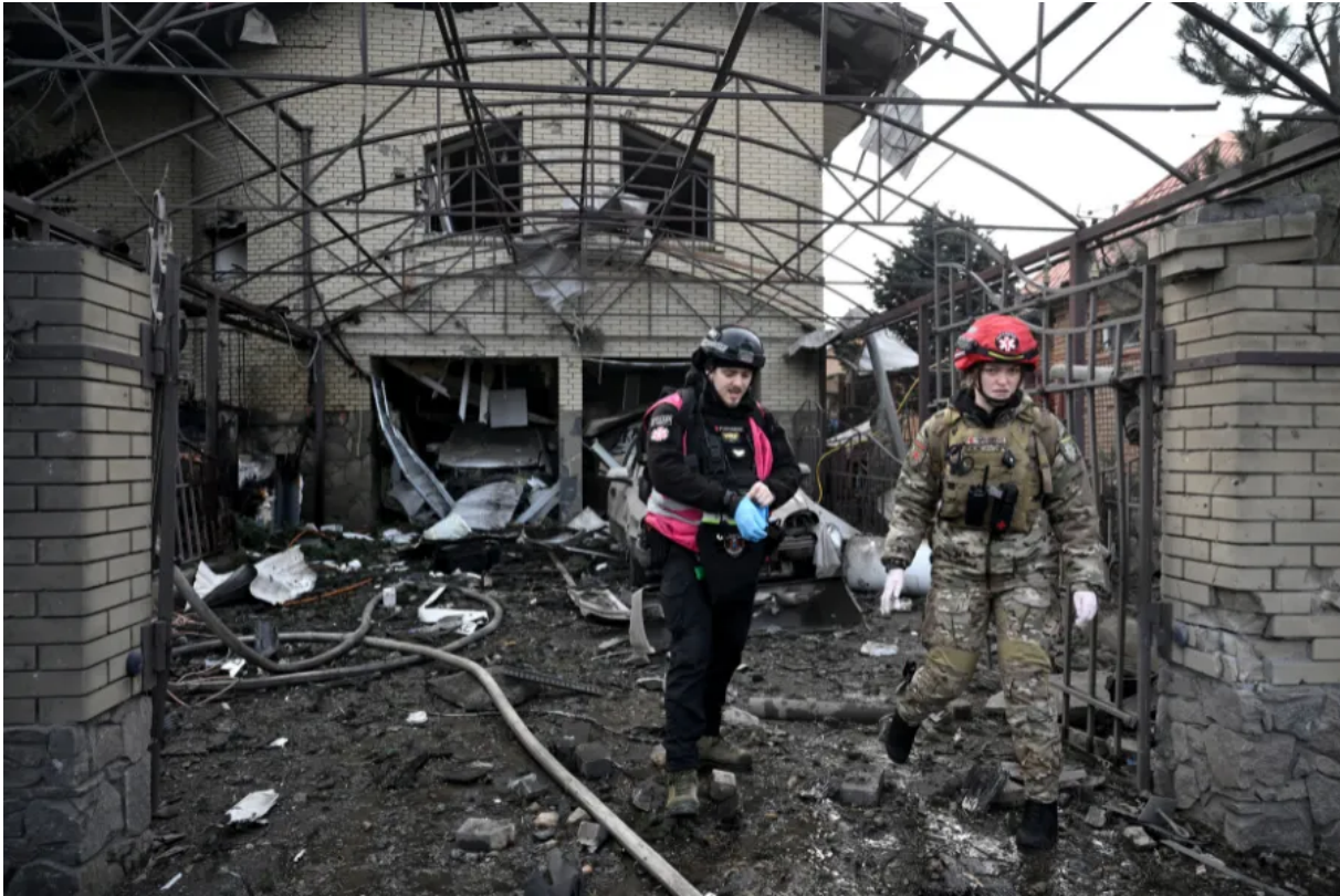
Paramedics walk over debris in front of a house and garage damaged by Russian bombing in Zaporizhia, Ukraine, on December 19, 2025. / Photo: DMYTRO SMOLIENKO / NurPhoto / NurPhoto via AFP
