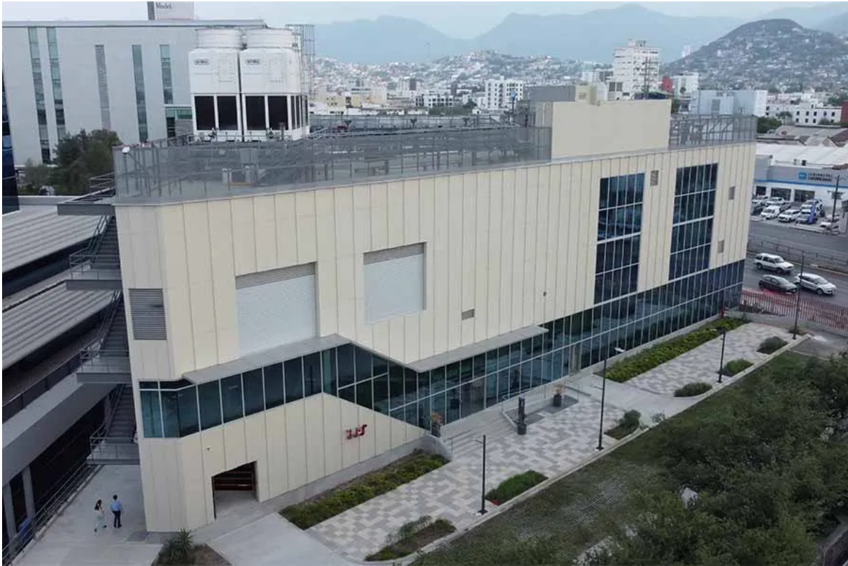
Núcleo is a District Power Plant that houses several energy generation systems. Photo: Jorge Valdés
